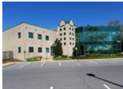
Dept of Rec & Park Headquarters Sep 2004-Sep 2011
