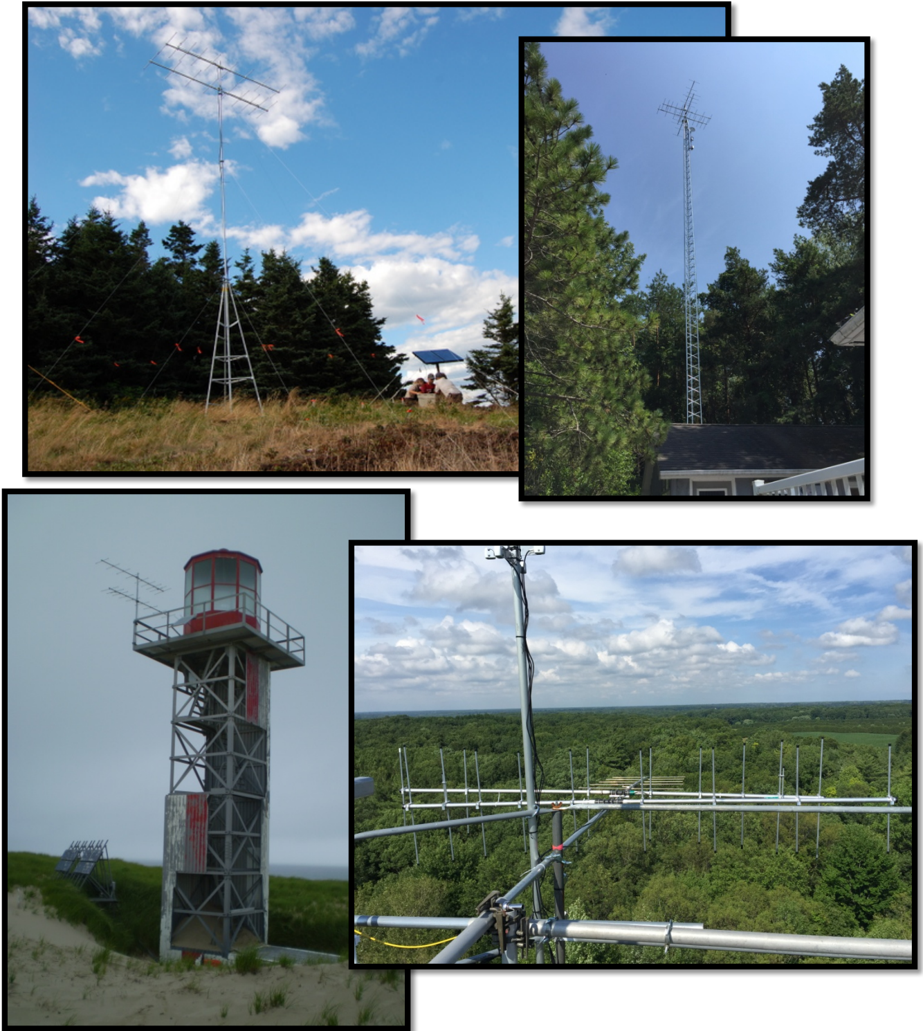
Figure 1. Examples of automated radio telemetry stations.
